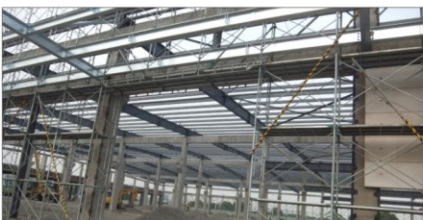
门式外墙脚手架的悬挑
